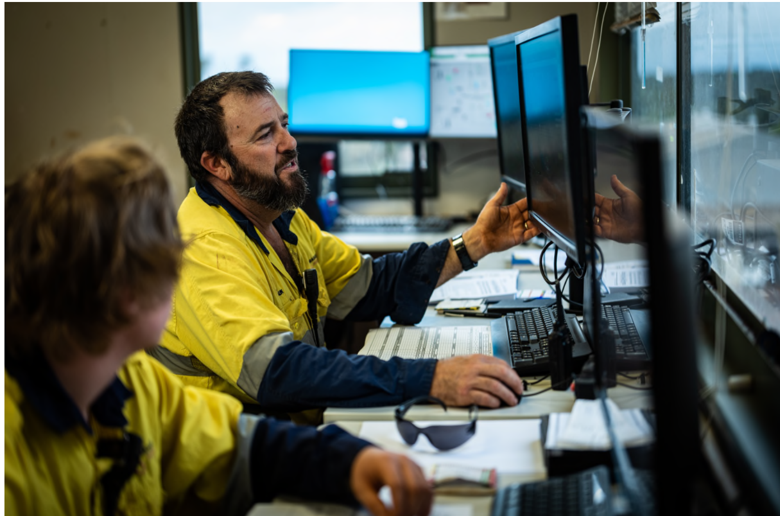
1.2Mtpa Davyhurst Processing Plant Control Room
